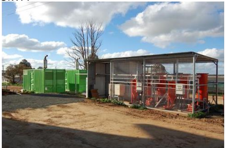
★ biogas gensets running in Australia poultry farm
